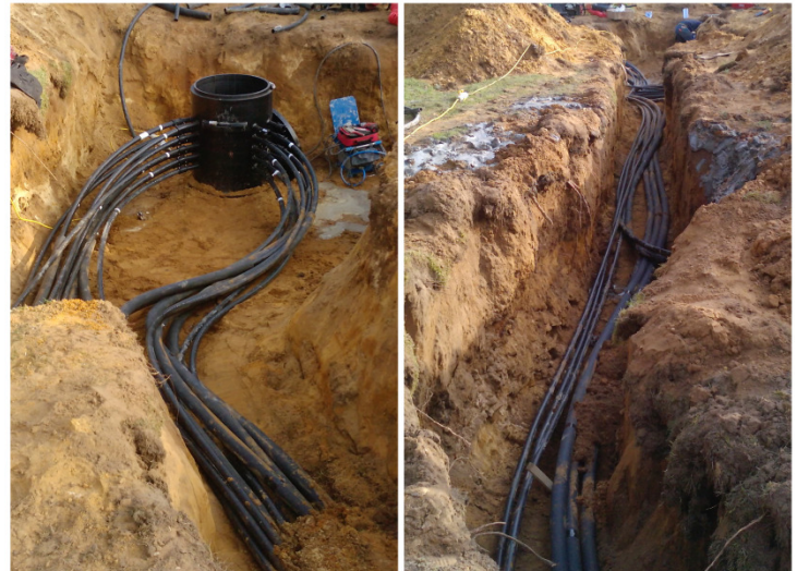
90 kW closed loop [borehole] GSH system
